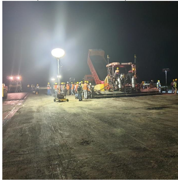
Reinstate pavement after concrete patch removal
