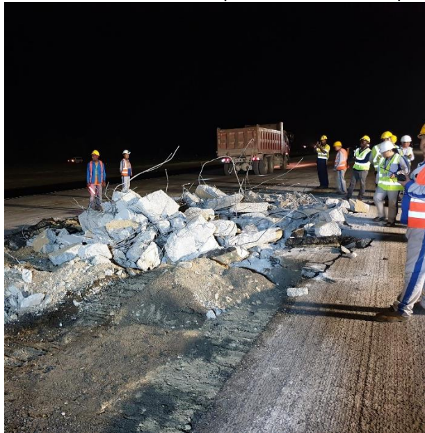
Removal of exist concrete patches – 400mm depth
